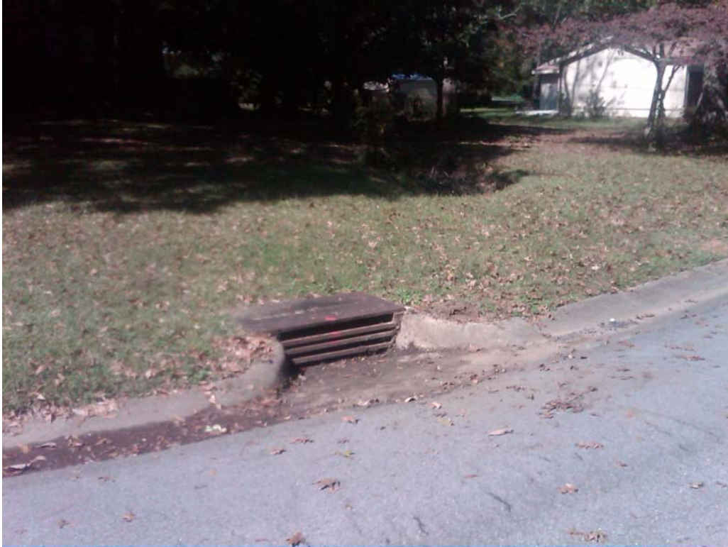
Photo 1 -- Inlet box at street in good condition
