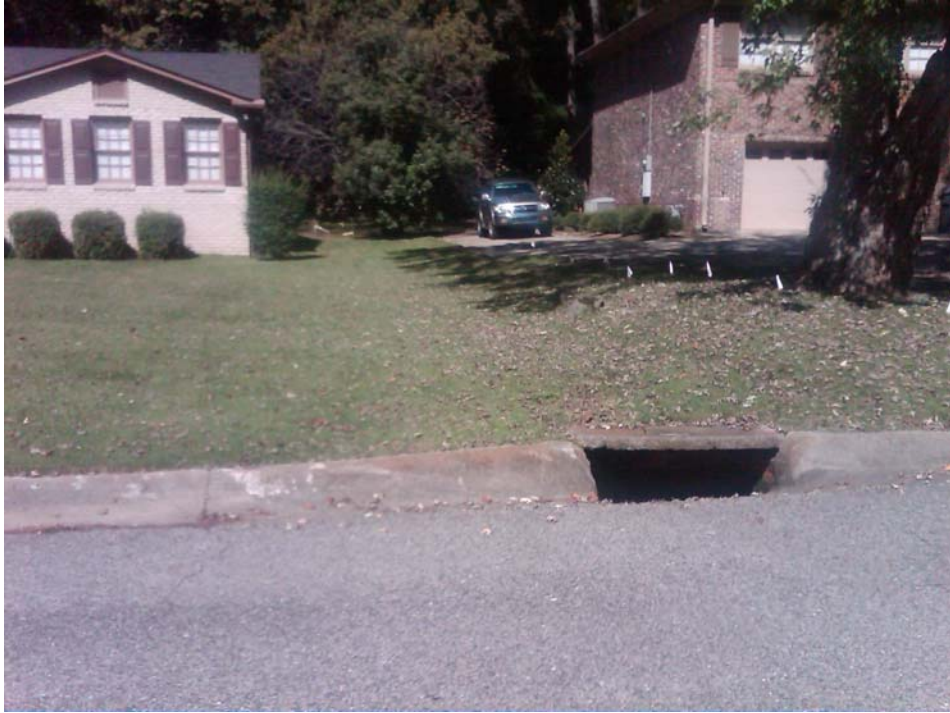
Photo 1 -- Drainage inlet box at road in good condition.
