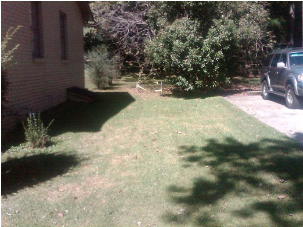
Photo 2 -- Sunken spots in grass area.
