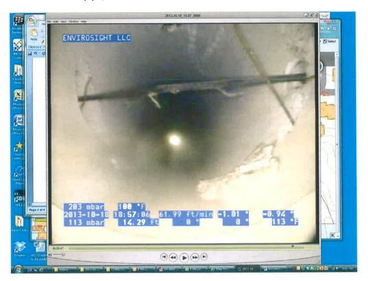
Photo 5: cable installed through walls of pipe
