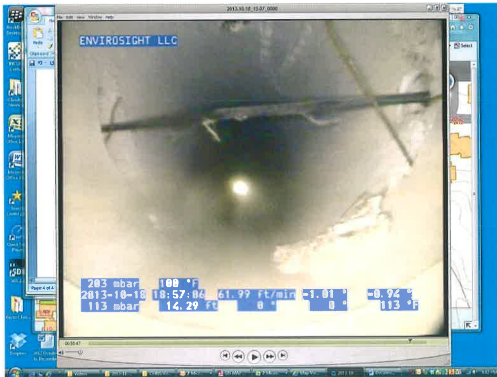
Photo 5: cable installed through walls of pipe
