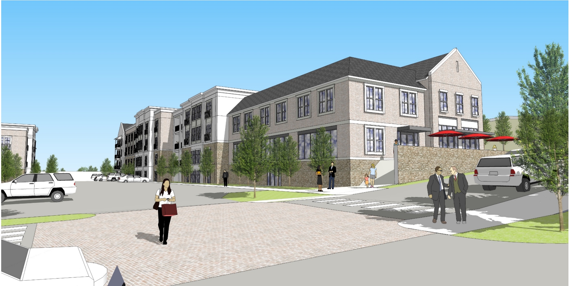
View looking southeast at back on Building #1
