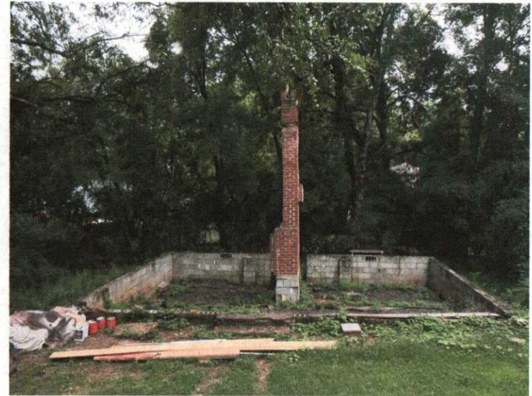
The foundation and chimney as they appear today, September 2015
