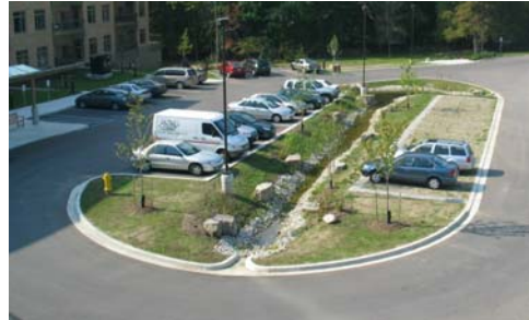
Recommended: Stormwater retention is incorporated into the site as a landscape amenity.
