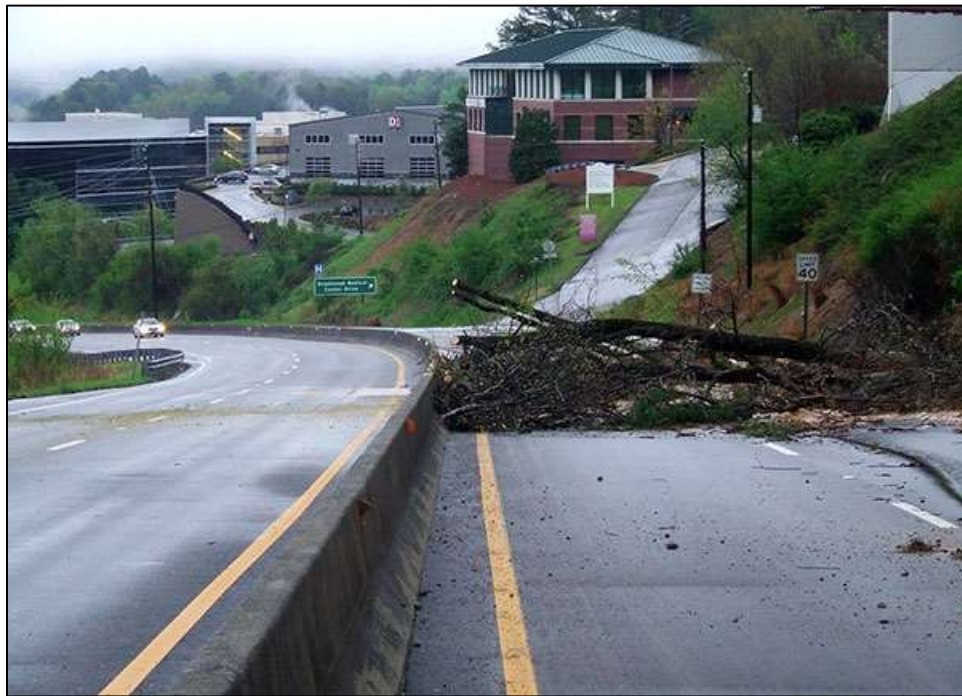
Image 4-1. Landslide at Highway 31 in Vestavia Hills
