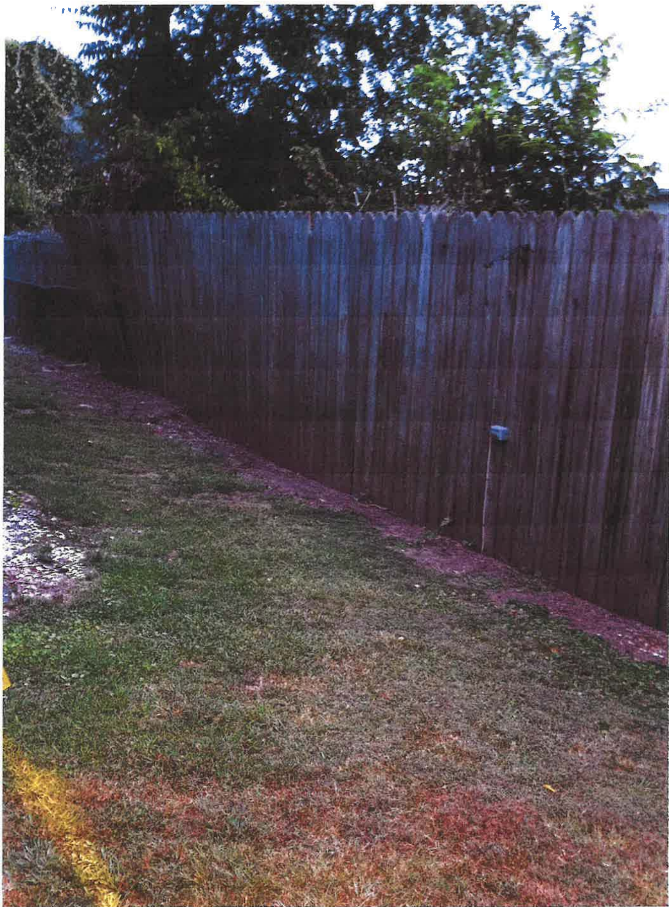
Previous 8ft Privacy Fence (Right side)
