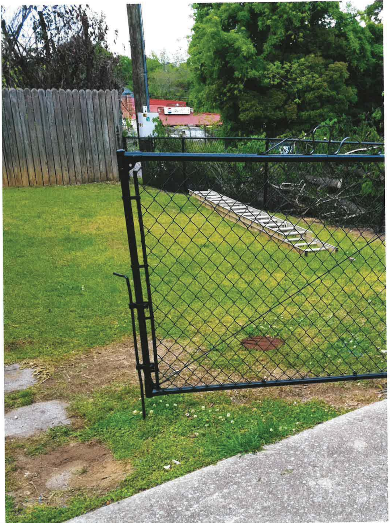
Previous 8ft. fence extending to the power pole in front yard. (Right side)
