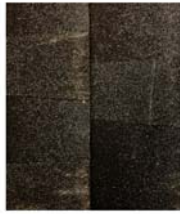
ASPHALT SHINGLE ROOFING
