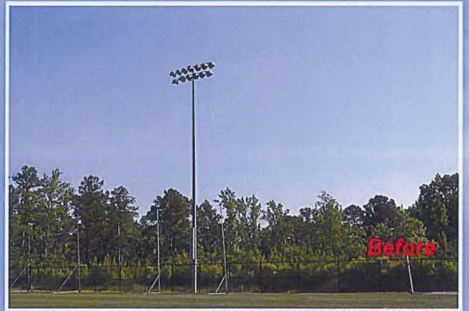
AT&T Liberty Park South Site (ID# 12778284 ) Vestavia Hills, Alabama 125-foot Light Pole Tower As viewed from Southwest
