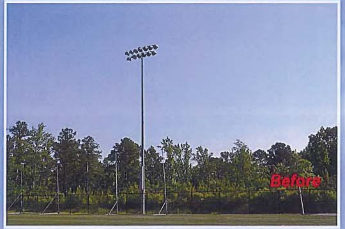
AT&T Liberty Park South Site (ID# 12778284 ) Vestavia Hills, Alabama 125-foot Light Pole Tower As viewed from Southwest
