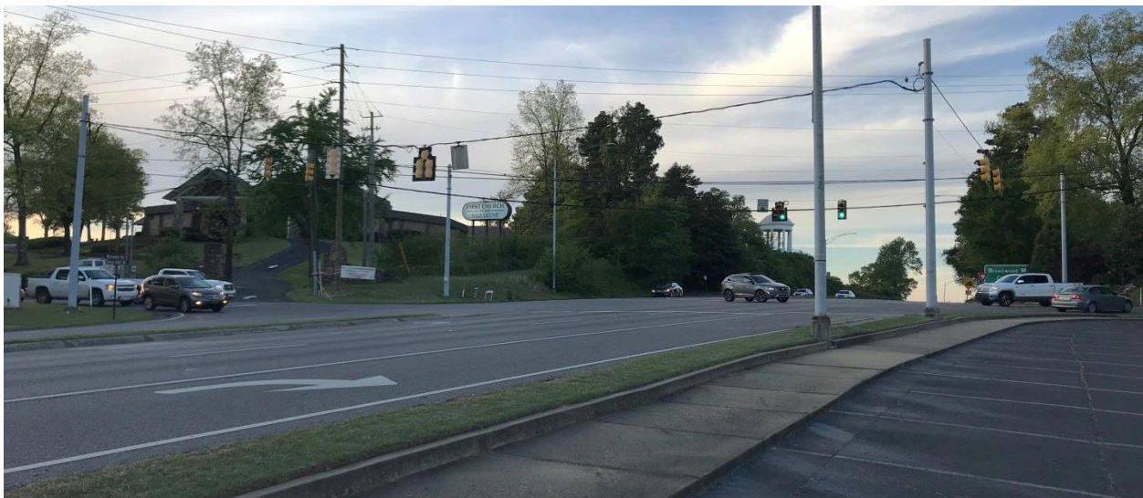
Figure 9: Looking north at the intersection of US-31 at Shades Crest Road
