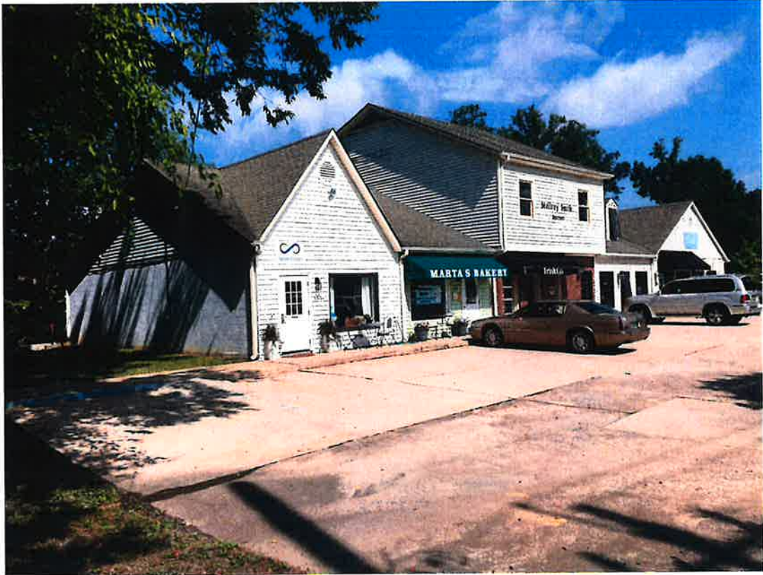
Existing building from the left side view
