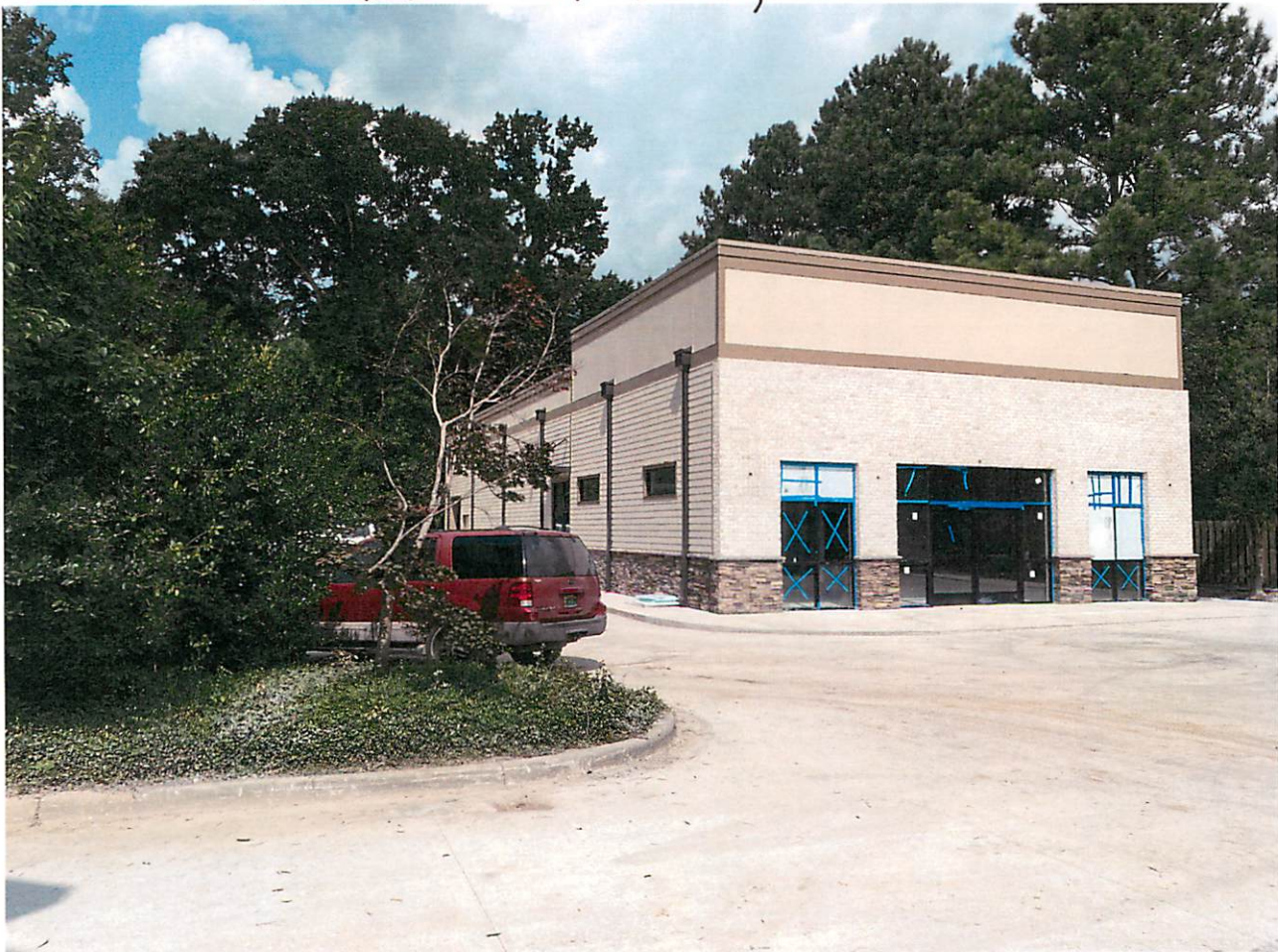
Front/side view of building ↗
