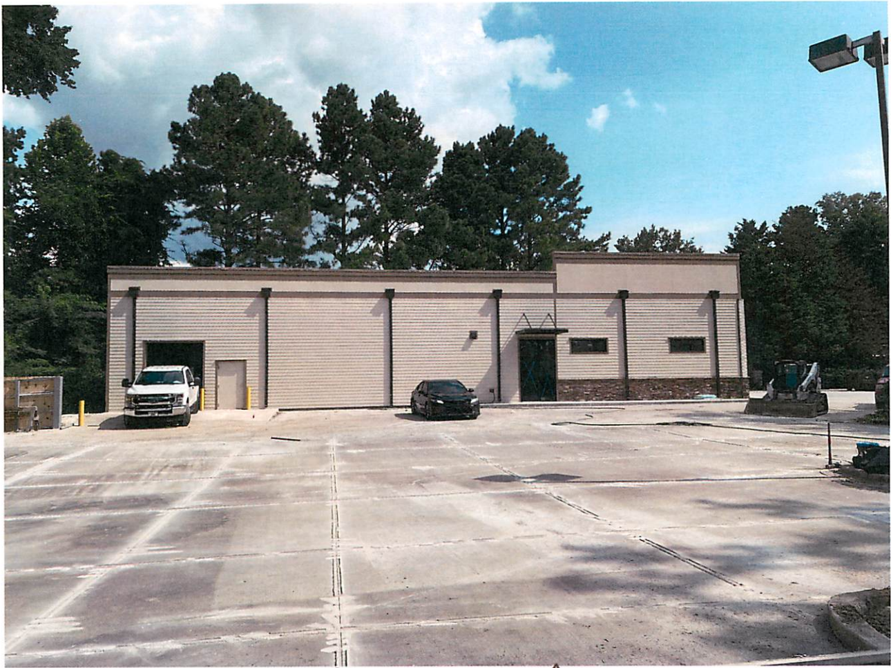
Side view of SW building ↗
