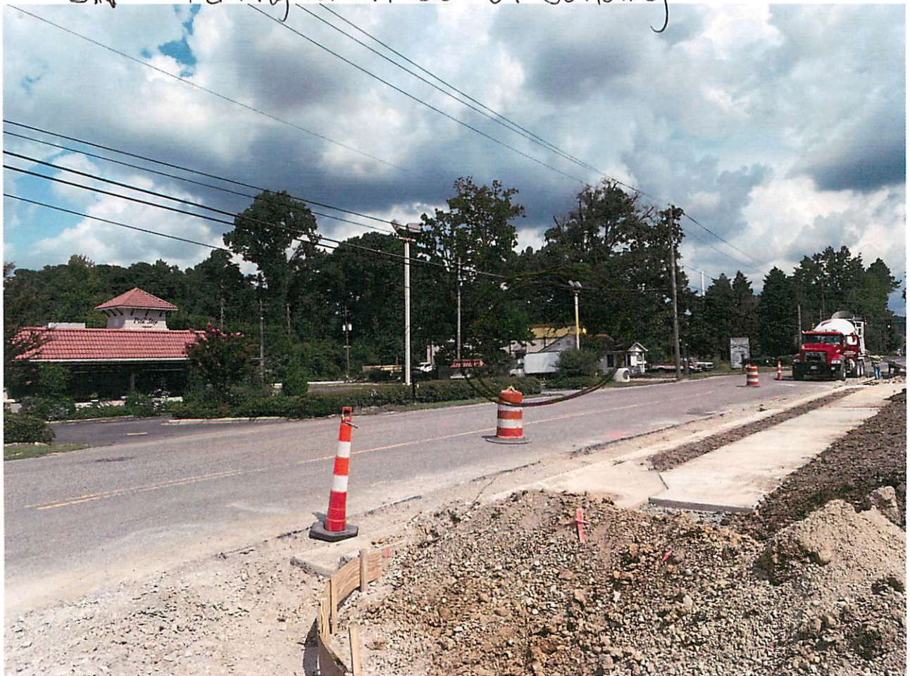
View of SW from Winn-Dixie entrance/Exit
