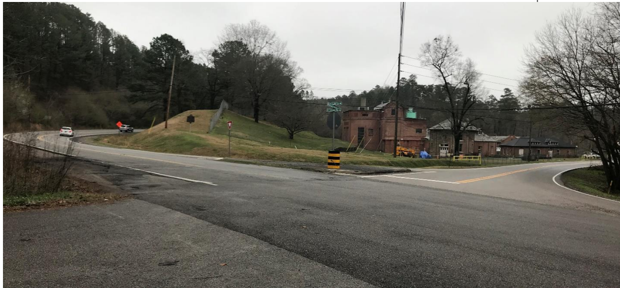
Photo 1: View of the Sicard Hollow Road at Blue Lake Drive/Cahaba Heights Road Intersection
