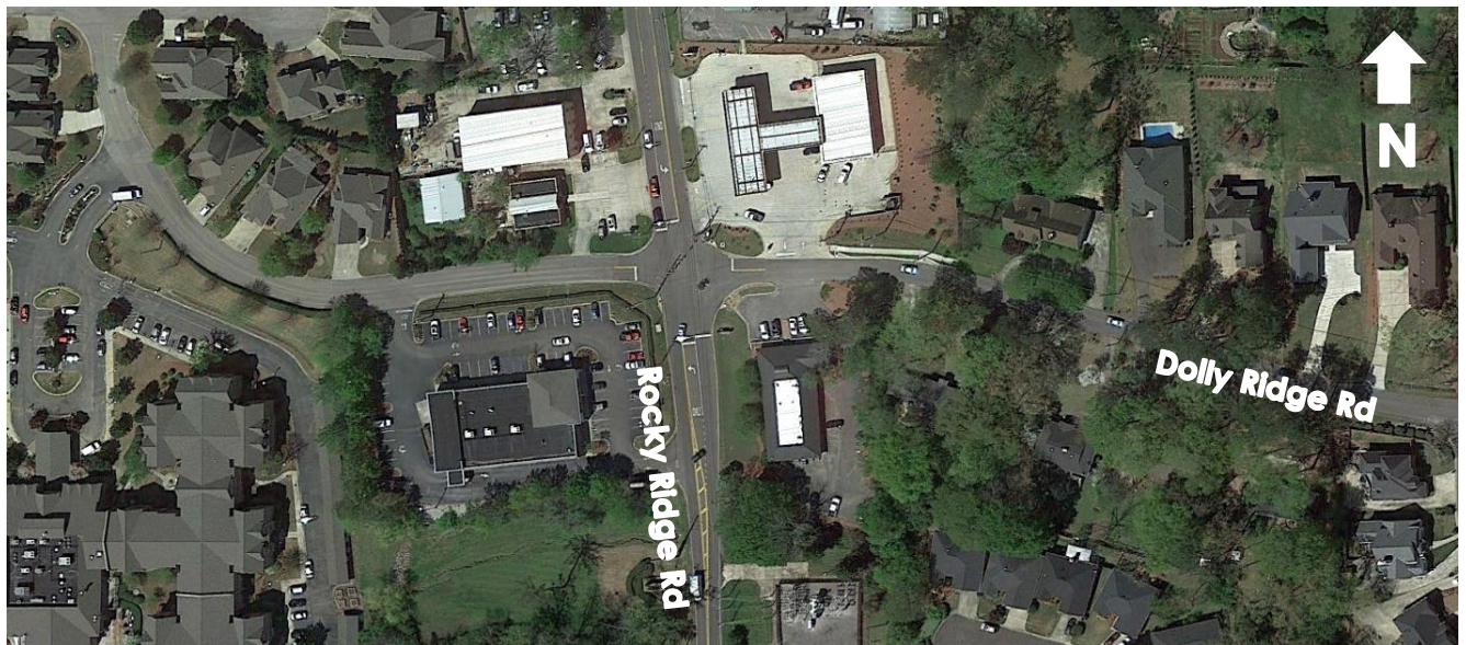
Figure 1: Aerial Imagery of the Rocky Ridge Road at Dolly Ridge Road Intersection
