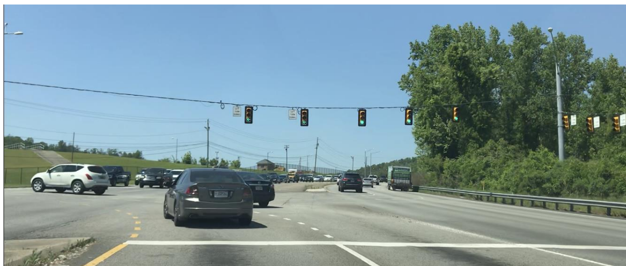
Figure 8: View of US-280 Westbound Left Turn Signal Heads
