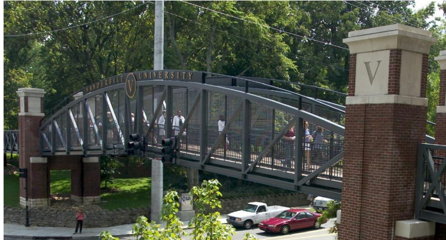
Figure 3: Vanderbilt University, Nashville, TN; Contractor: Centex Rodgers, Inc.; Truss Supplier: Contech
