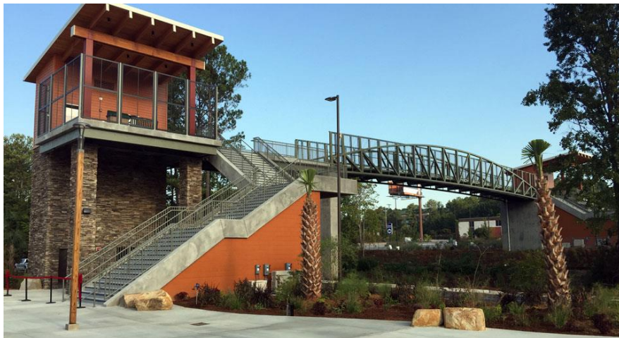
Figure 1: Riverbanks Zoo Expansion, Columbia, SC; Contractor: Rodgers Builders; Truss Supplier: Contech
