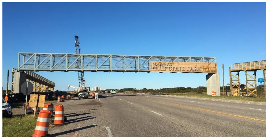
Figure 2: Front Beach Rd, Gulf Shores, AL; Contractor: Banner Industrial Construction, Inc.; Truss Supplier: Qualico Steel
