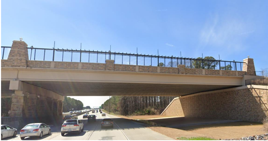
Figure 7: Encore Parkway Bridge, Alpharetta, GA using Blub-Tee Girders; Image from Google Earth
