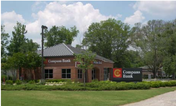
Existing commercial development on Crosshaven Drive
